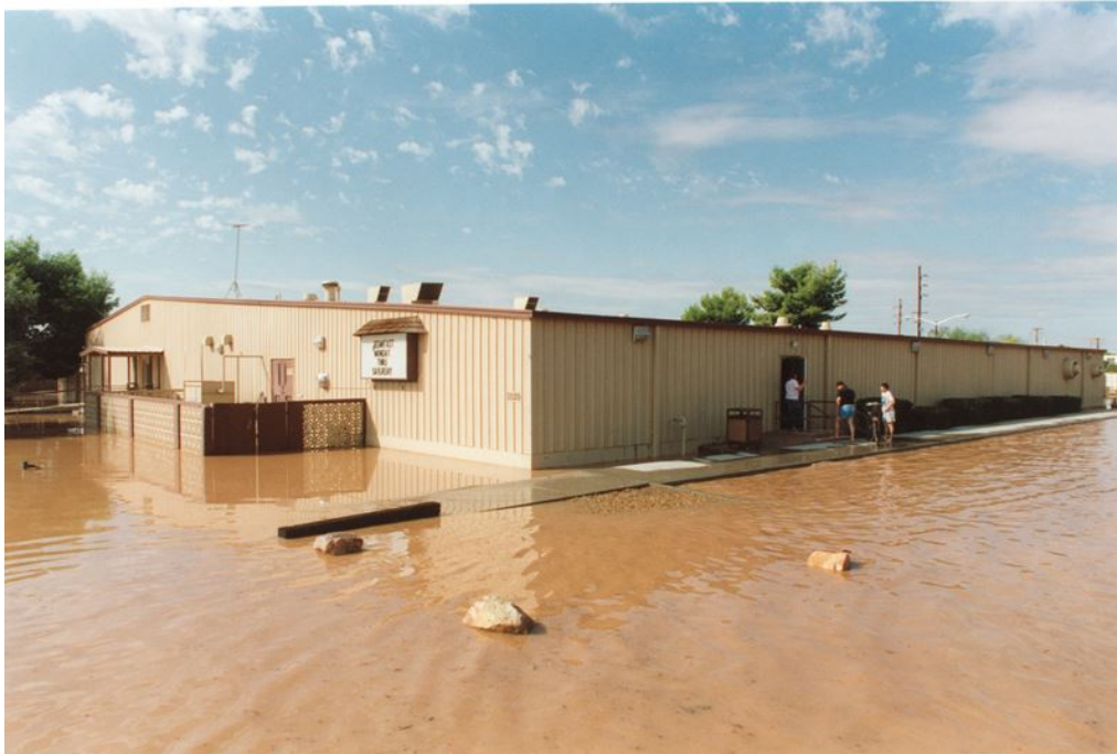
Flooded Base Bowling Alley, 20 October 1992
