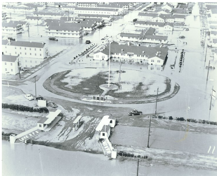
Flooded Front Gate
